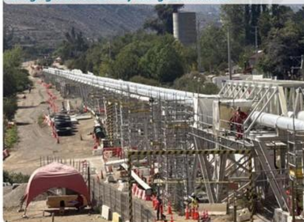
New concentrate pipeline (March 2026) Bridging work underway along 120 km route
