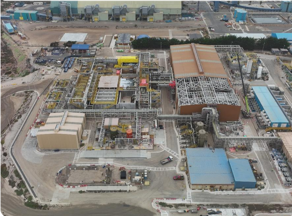
Desalination plant expansion (March 2026) Construction of seawater reverse osmosis building
