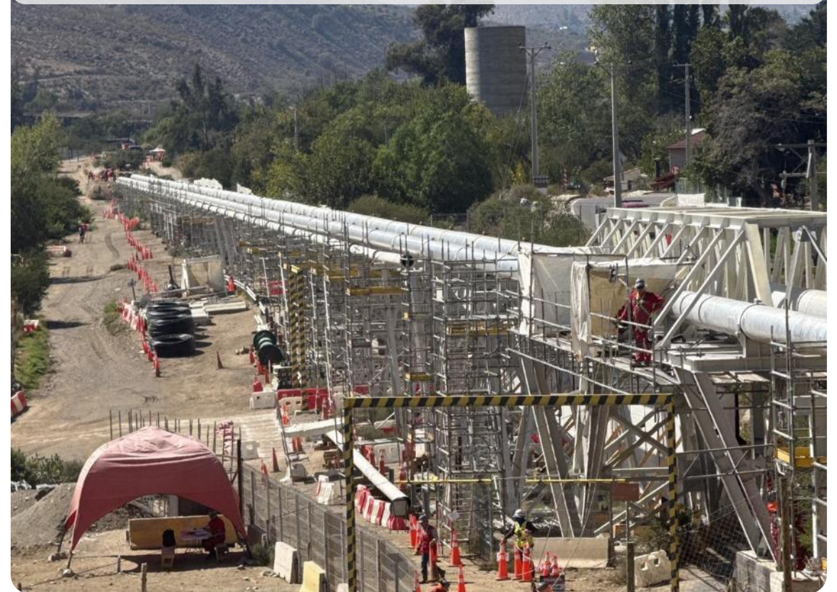
New concentrate pipeline (March 2026) Bridging work underway along 120 km route
