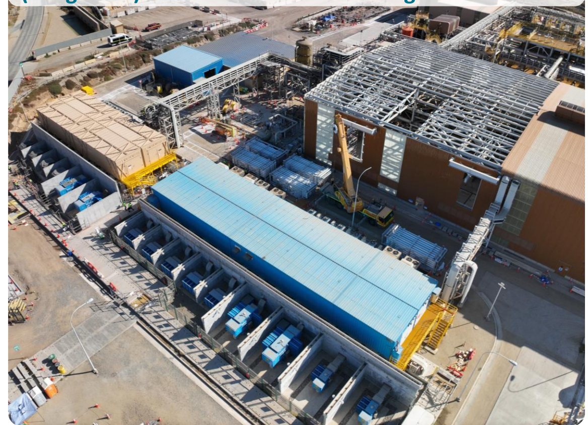
Desalination plant expansion: Pump installation (foreground) and reverse osmosis building
