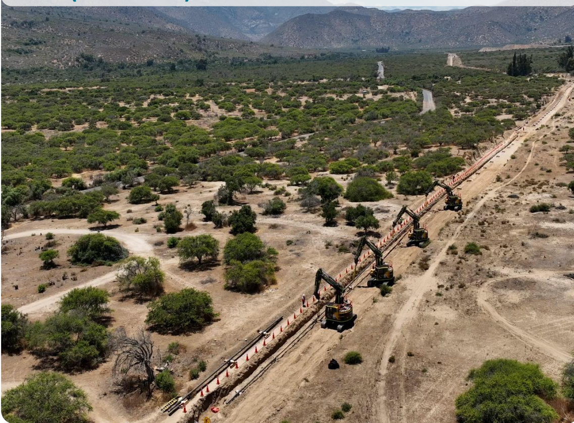
New concentrate pipeline: Installation work along 120 km route (low section)
