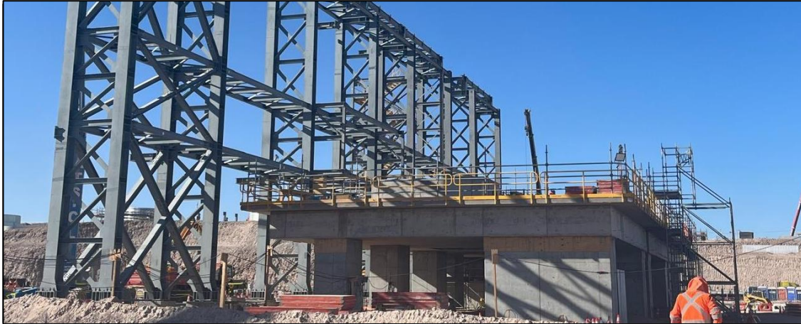
Image: Foundations and steel structure to house tertiary crushers, main concentrator site
