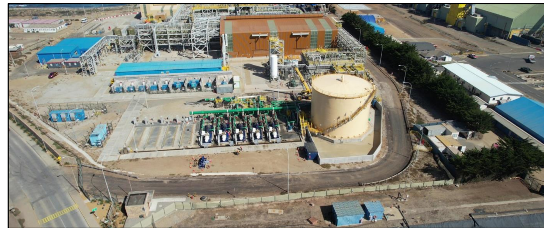
Image: Desalination plant – concrete pad with existing pumps (right) and space for expansion (left)
