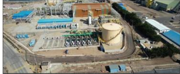
Image: Desalination plant – concrete pad with existing pumps (right) and space for expansion (left)
