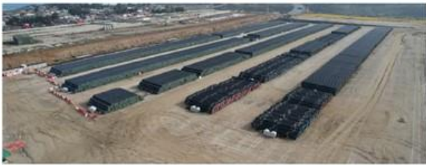
Image: Concentrate pipeline – stockyard ahead of pipeline installation along new route
