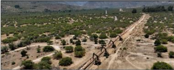
Image: Concentrate pipeline – cranes installing the new pipeline along the lower section
