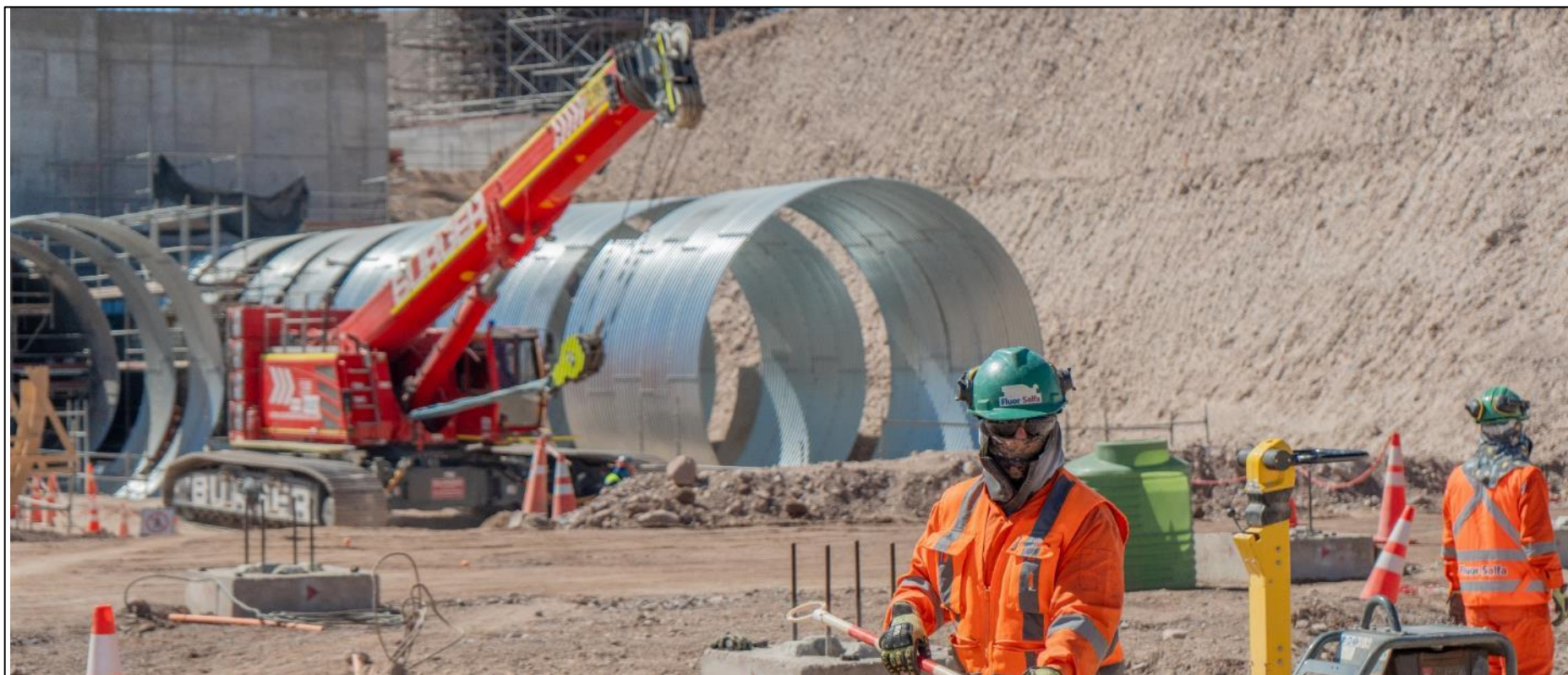
Image: Installation of ore rehandling tunnels, main concentrator site
