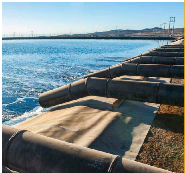
Seawater storage reservoir at Antucoya.
