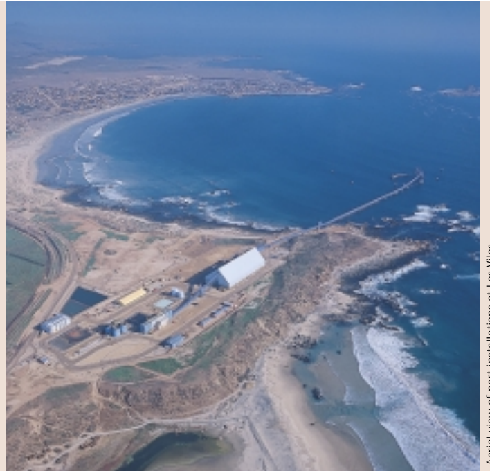
Aerial view of port installations at Los Vilos
