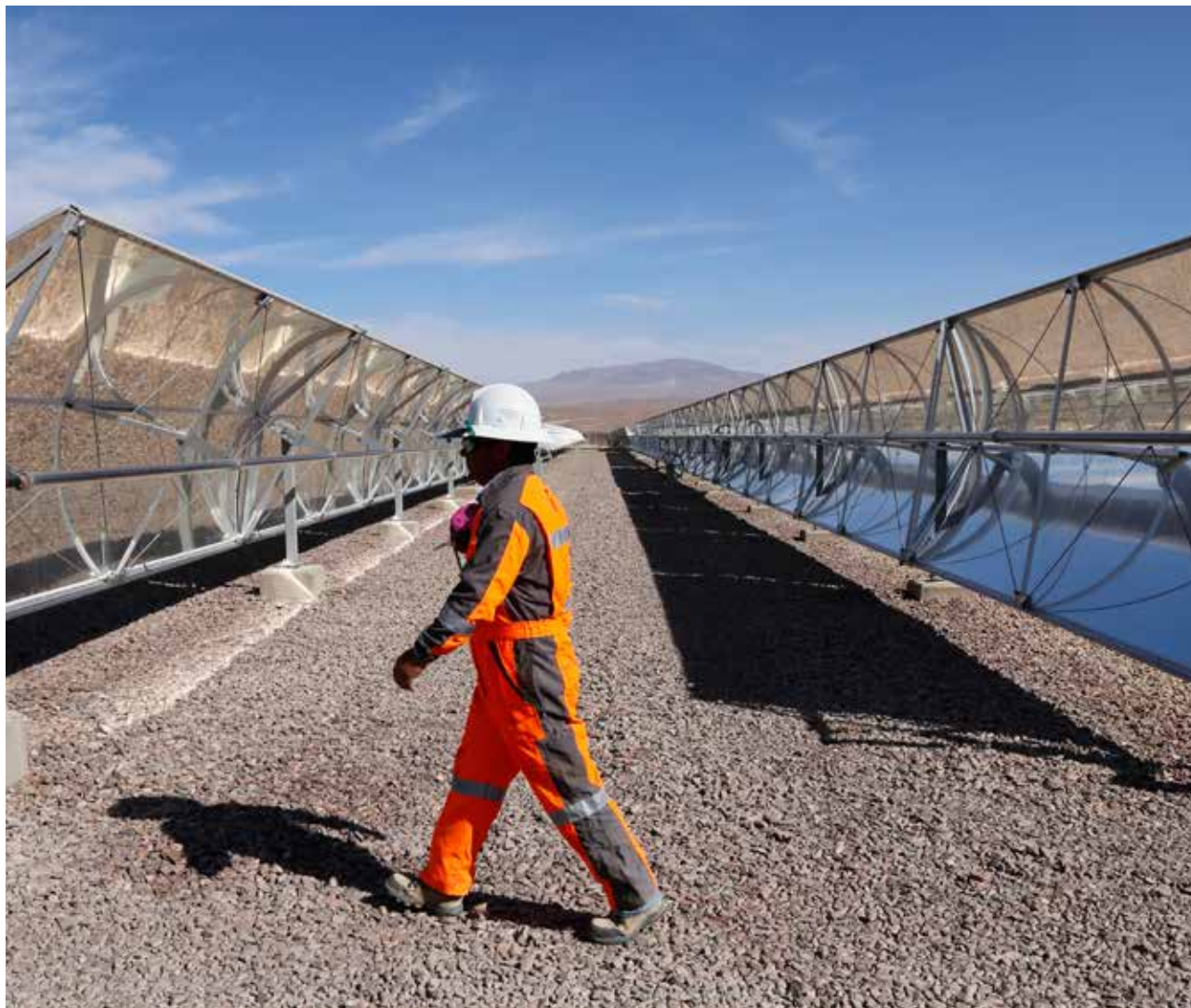
Centinela solar power plant.
