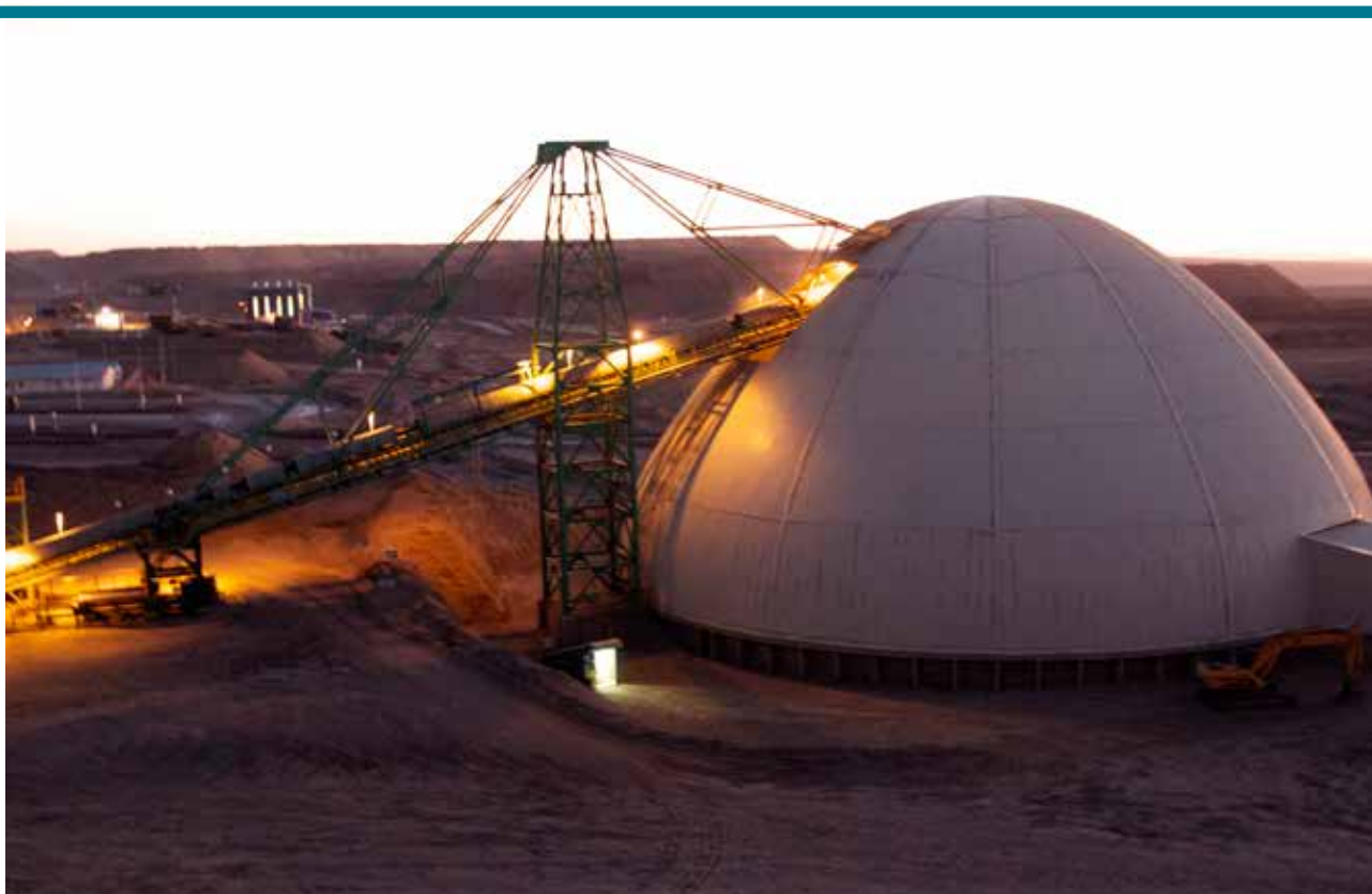
The stockpile dome at Centinela was completed in 2014.
